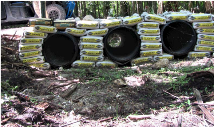
This was one of the many culverts replaced during the culvert project on West Main in May of 2020.
